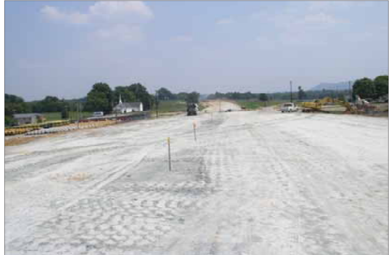
currently under construction
